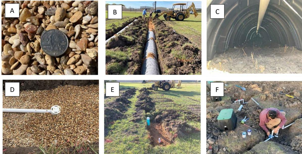
Figure 8. Images of the installation process: A) pea gravel, B) Leaching chamber installation, C) Location of lateral under leaching chamber, D) Orifice shields in gravel trench, E) Closing of a gravel trench, showing inspection port and valve, F) Connection of laterals to manifold
