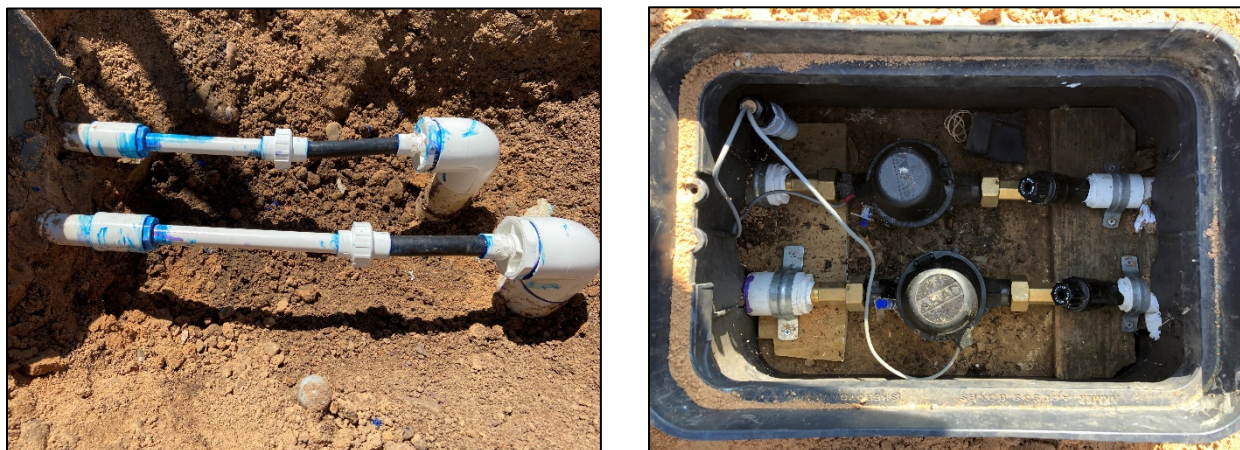
Figure 10- a) Restricted orifice flow regulators, b) electronic flow meters
