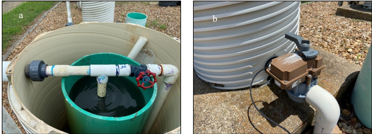
Figure 7- a) ATU influent metering reservoir, b) automated valve.
