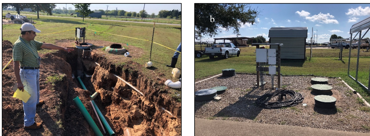
Figure 6- a) RELLIS sewer line and Lift Station, b) OSSF Feed Tank
