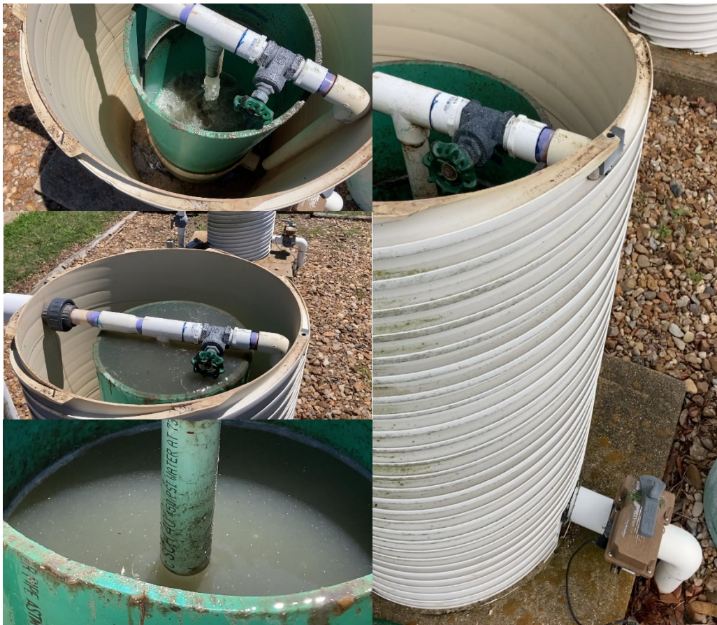
Figure 17. Calibration tank phases. Left top: loading; Left center: draining surplus; Left bottom: calibrating (loading ended); Right: Jandy valve open to send calibrated volume to the septic tank
