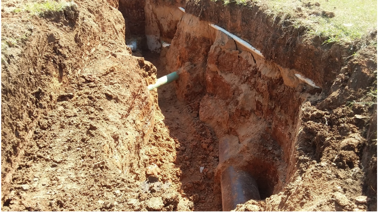
Close-up of the clay sewer line in the area where it will be tapped in for connection to the lift station.
