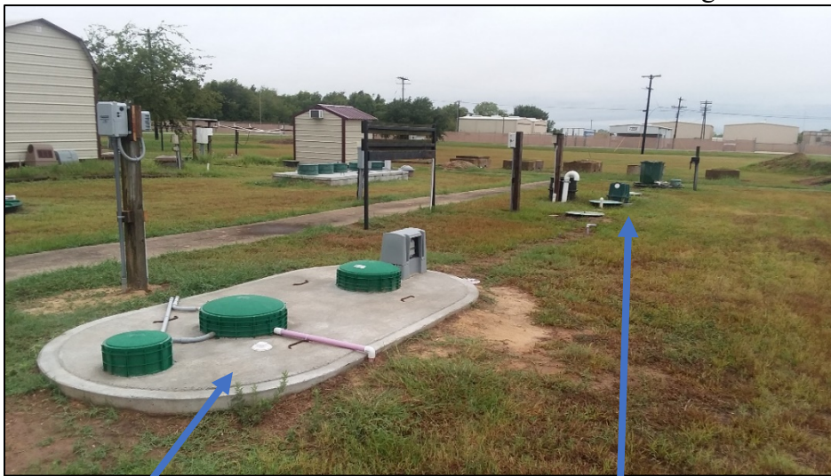
Cleatstream 500-DA reuse treatment tank and BioBarrier MBR 0.5 tank
