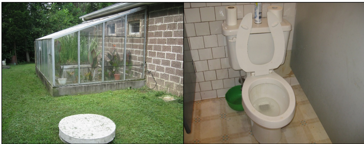
Photo 10: Wetland in a climate-controlled greenhouse on-site wastewater treatment system for a community center in Virginia. Treated wastewater is disinfected using UV and polished using an inline charcoal filter just before reusing it for toilet flushing.
