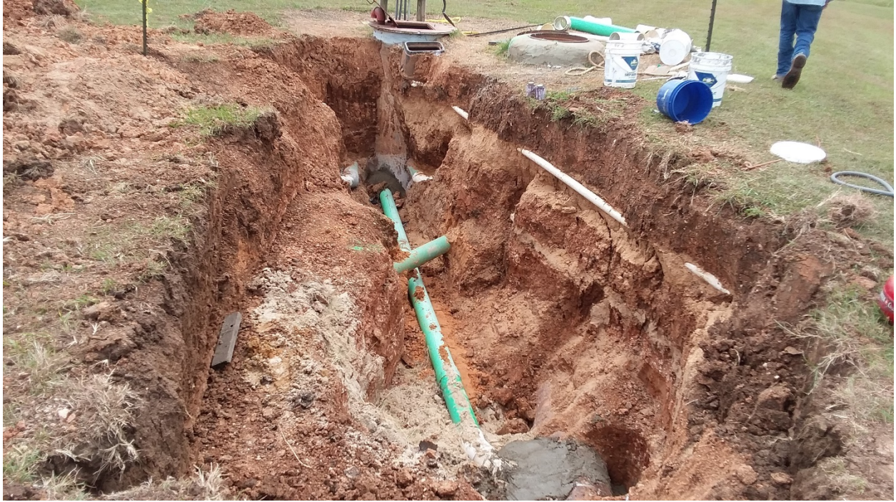
Sewer line connected to the lift-station using a 4-inch gravity sewer pipe (green color pipe).
