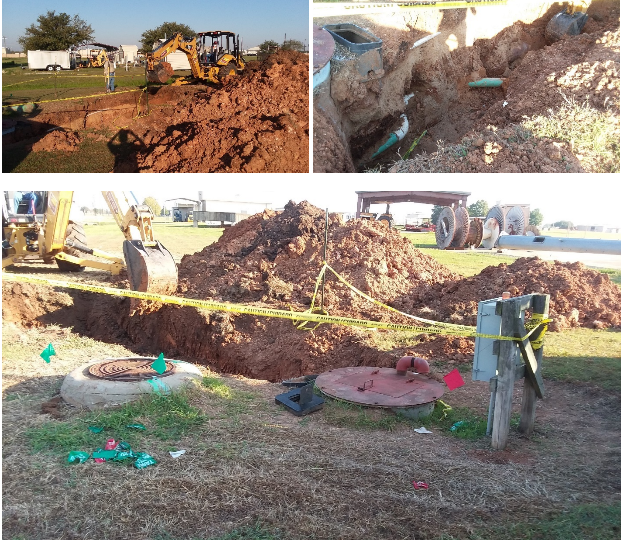
Top Left: Excavation work to expose underground pipe network; Top Right: Underground pipe network, clay pipe is the main sewer line and other PVC pipes are connections between the lift-station and the feed tank. Bottom large picture shows above ground conditions, concrete manhole (on left) and the fiberglass lift-station (on right).
