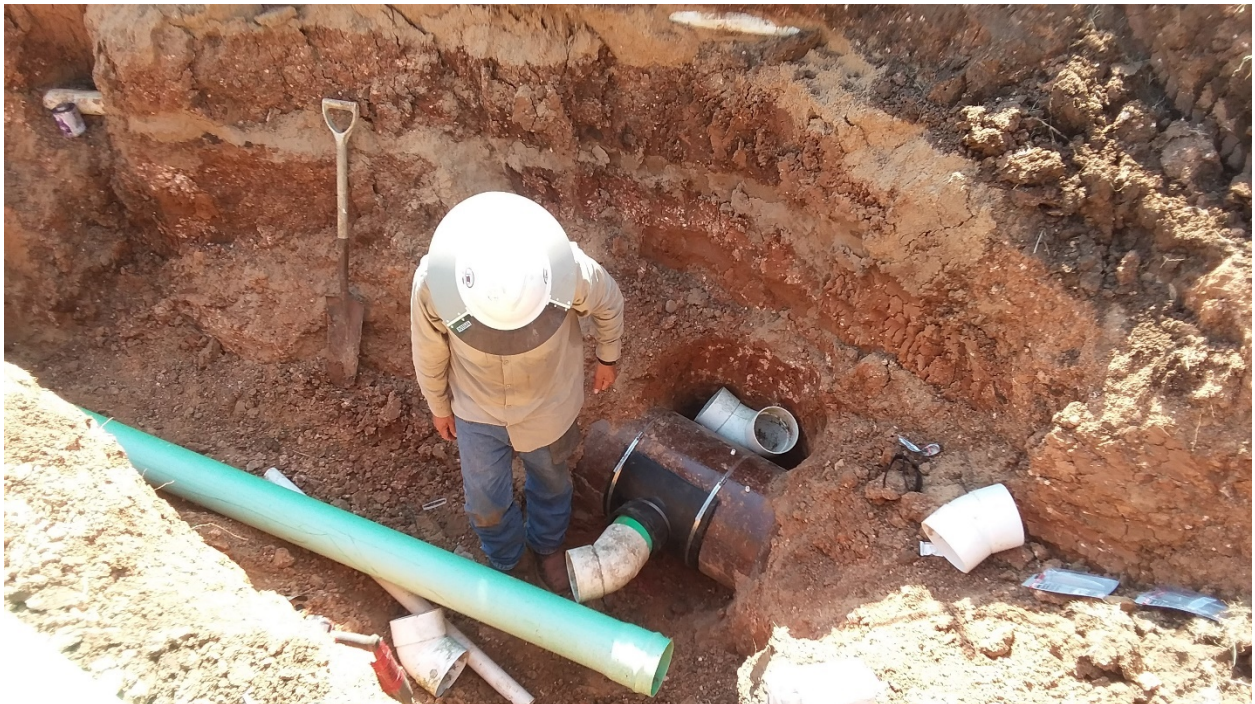
Creating the connection between the clay sewer line and the manhole using a 4-inch gravity sewer line (green color pipe).
