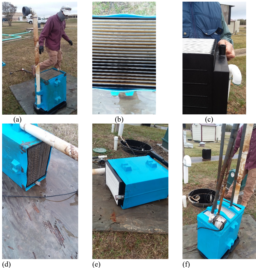
Photo 4: (a) removal of the old membrane cassette from the MBR-aeration tank; (b) close-up of membrane fouling (about 18 months in use); (c) close-up of the new membrane cassette that will replace the old one; (d) carefully draining wastewater from the old cassette, (e) replacing the old cassette with the new one, and (f) re-assembling the membrane unit for putting it back in the MBR aeration tank; difficult work that must be done by a trained person with at least one helper
