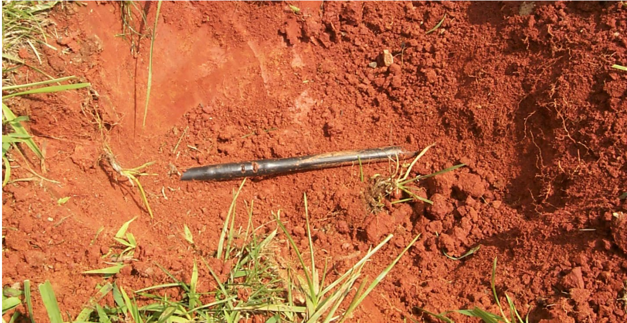
Figure 6. Drip dispersal following ATU unit working correctly (about 4.5 years in use).
