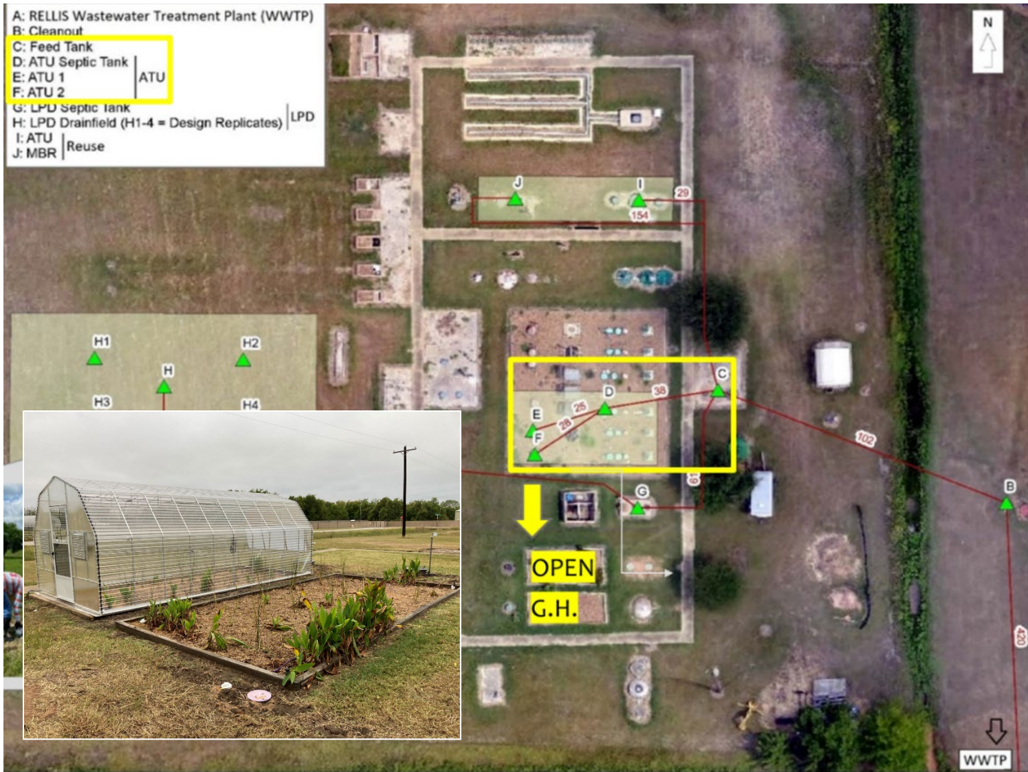
Figure 16. Aerial view of the TAMU OSSF Center. Features C, D, E, and F were used for the experiment. Drip lines were laid out in two wetlands (“OPEN”, open wetland, and “G.H.”, greenhouse). A lateral view of the two wetlands is also shown.
