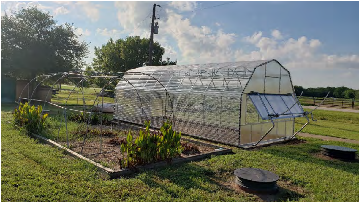
View from the back end of the Greenhouse, note the large window at the back end has an adjustable opening mechanism to control the air flow through the Greenhouse.
