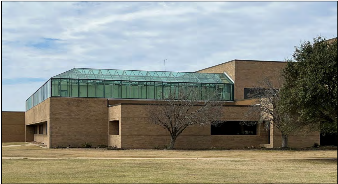
Building #1516, one large greenhouse on roof top
