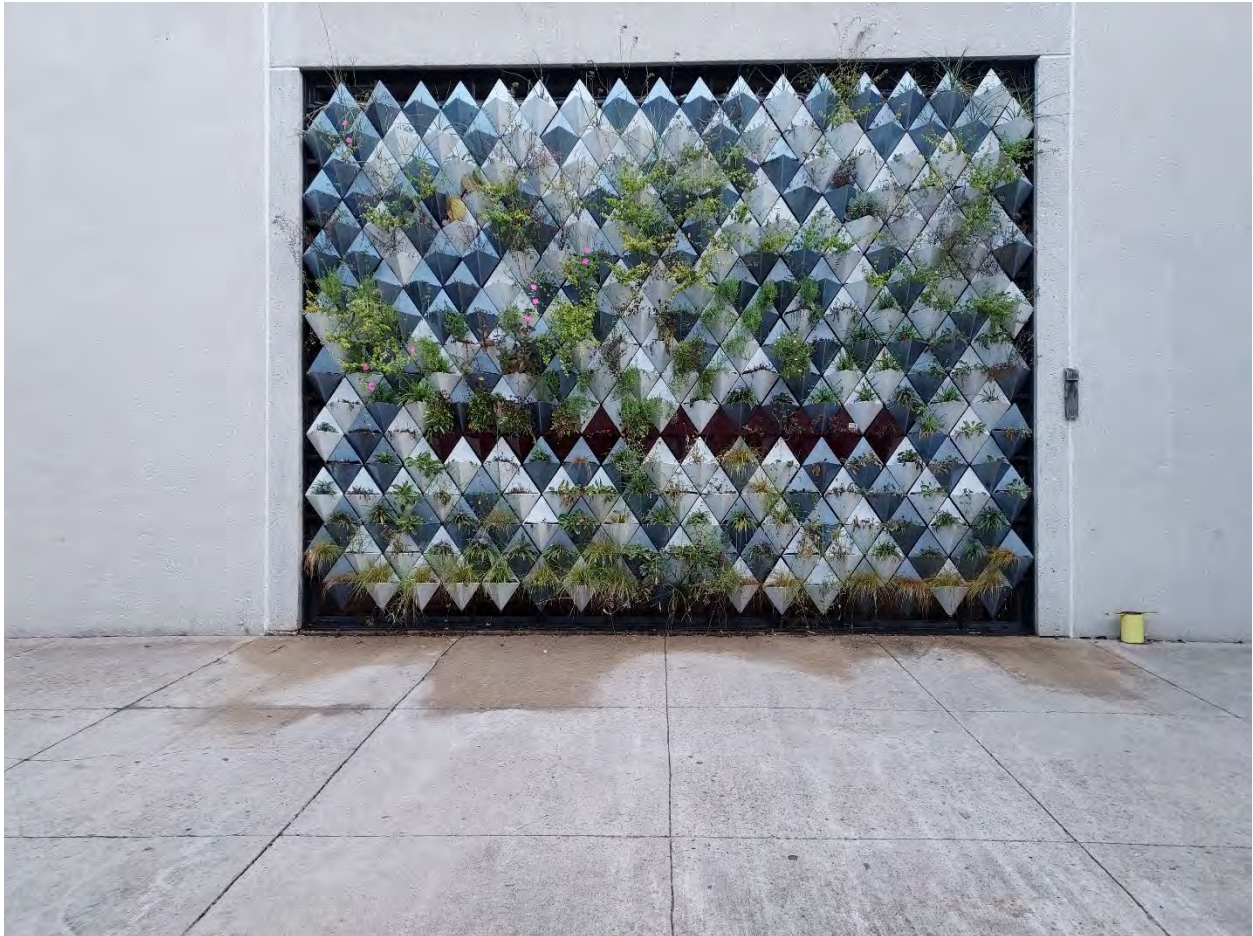
Green Wall operating on TAMU Main Campus, showing wetness indication of excess irrigation (September 7, 2022)
