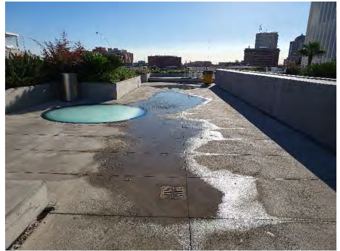
The Green Roof covering about one-acre space, and big wet spot indicating over irrigation and/or lack of ET losses.
