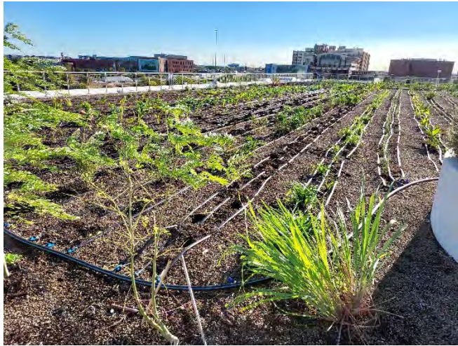
The Green Roof covering about one-acre space, and big wet spot indicating over irrigation and/or lack of ET losses.
