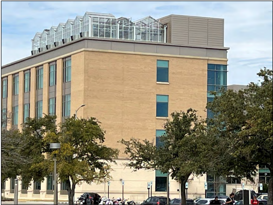
Building #1515, multiple greenhouses on roof top
