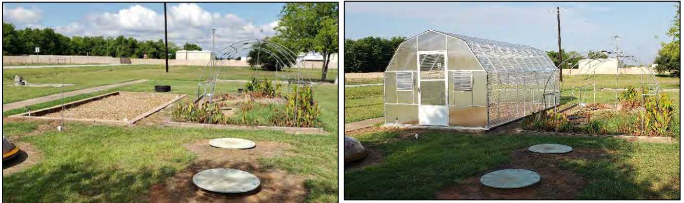
Photo 5: Wetland cells before (L) and after installation of the Greenhouse (R)
