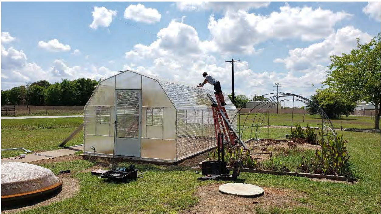
11x24 Big Barn Greenhouse installation day.
