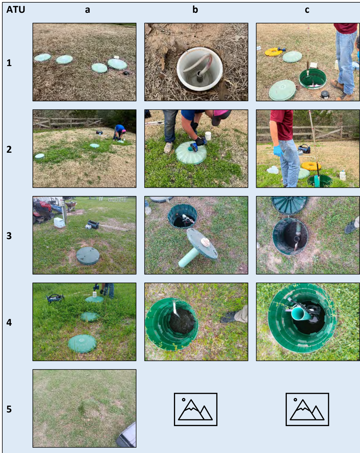
Plate 1 – Photographs of ATU systems 1 through 5. Designations a, b, and c generally show a) overall system, b) pump tank, chlorinator, or lid condition or other anomaly, and c) sludge condition (if available).
