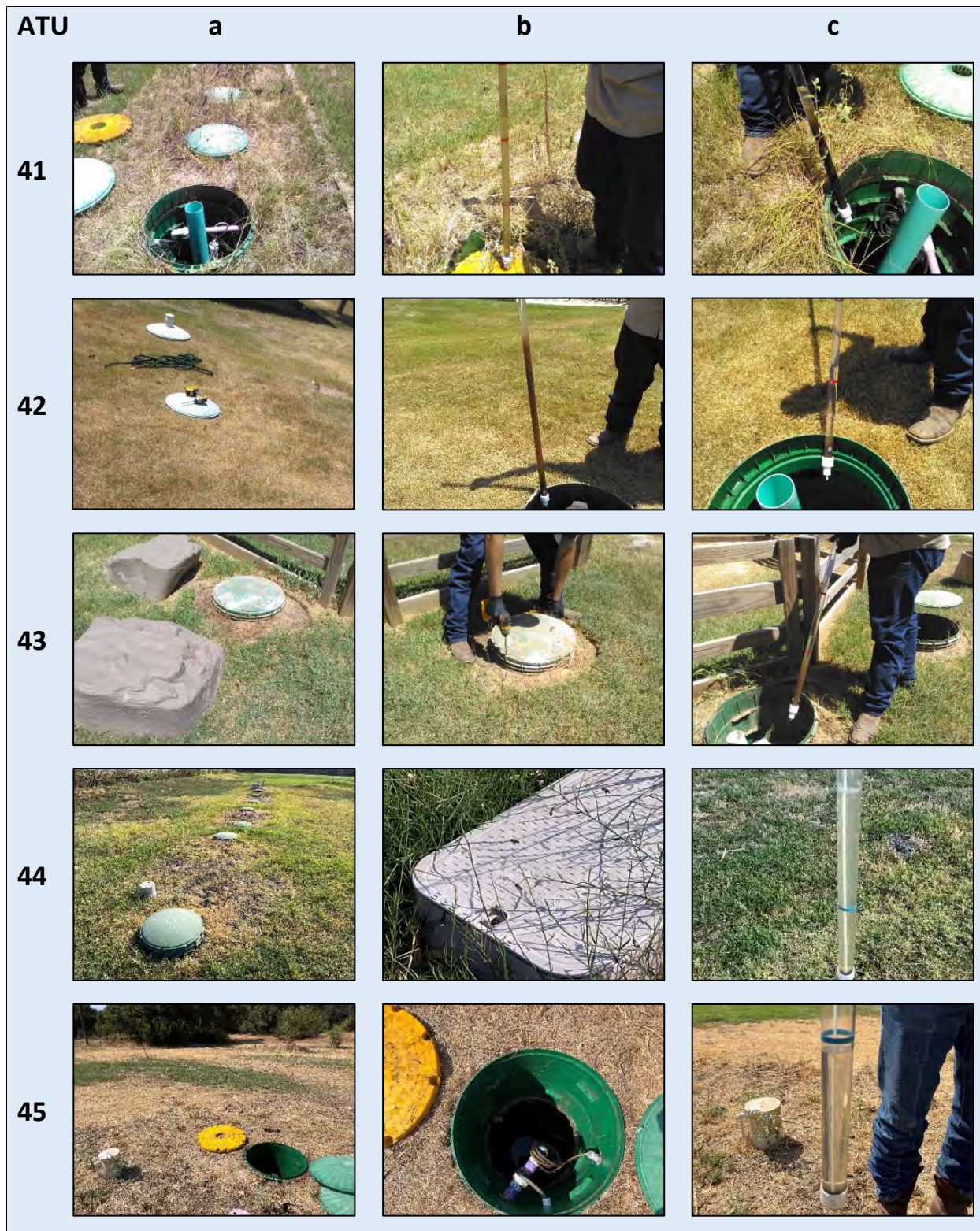
Plate 9. Photographs of ATU systems 41 through 45. Designations a, b, and c generally show a) overall system, b) pump tank, chlorinator, or lid condition or other anomaly, and c) sludge condition (if available).
