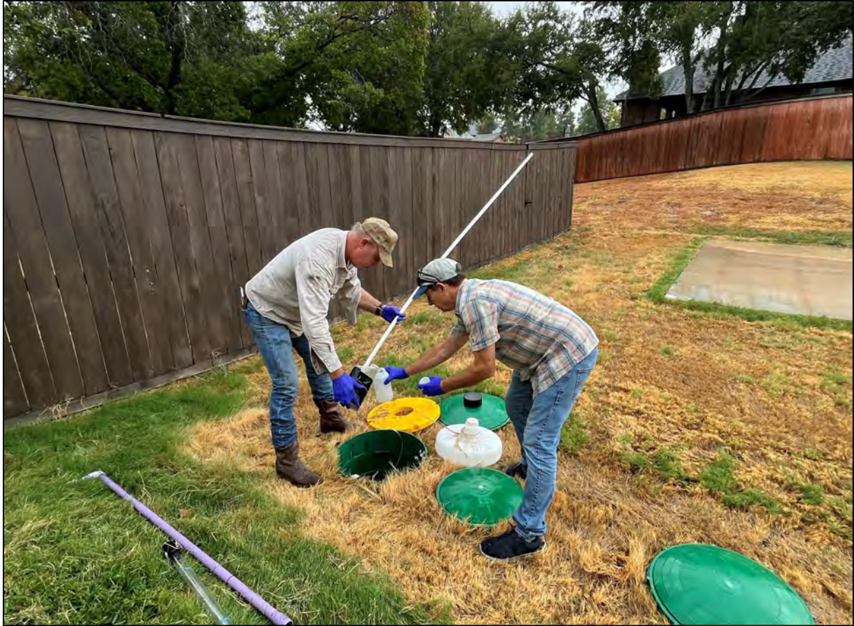
Figure 6- Collecting water quality sample from ATU pump tank.
