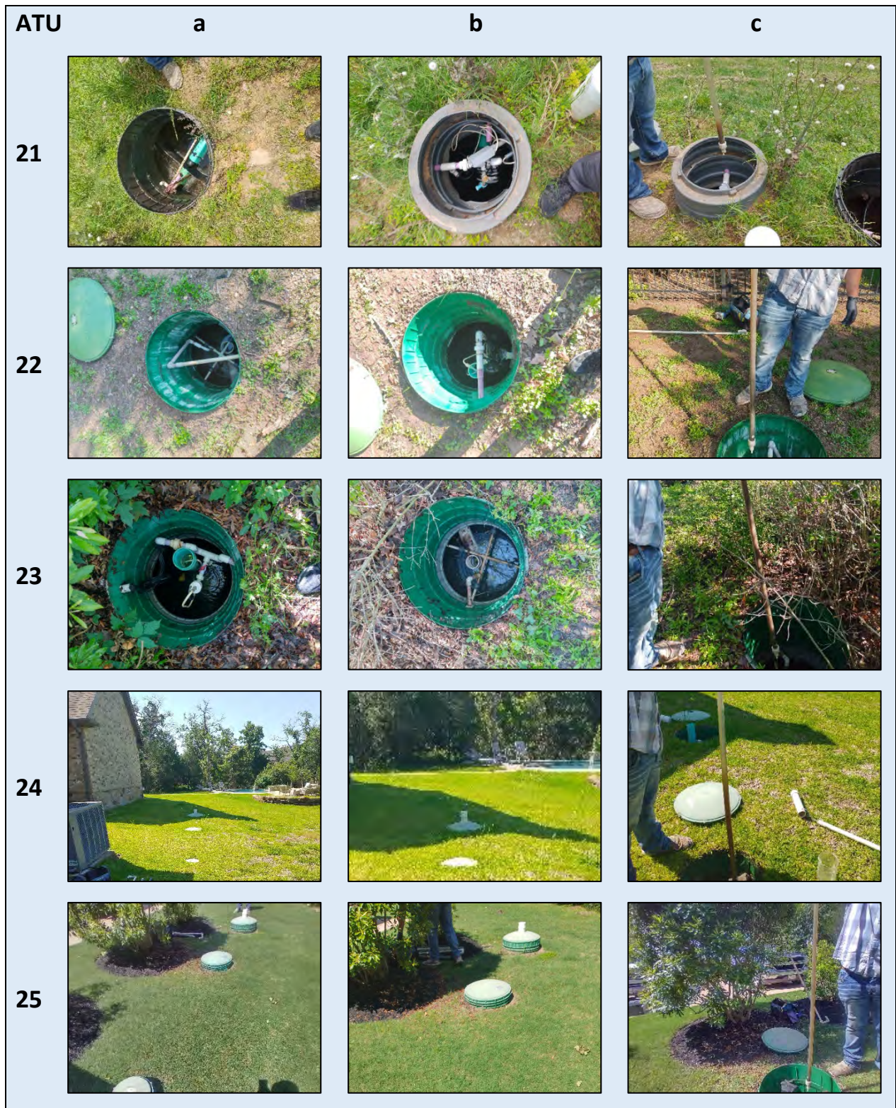
Plate 5. Photographs of ATU systems 21 through 25. Designations a, b, and c generally show a) overall system, b) pump tank, chlorinator, or lid condition or other anomaly, and c) sludge condition (if available).
