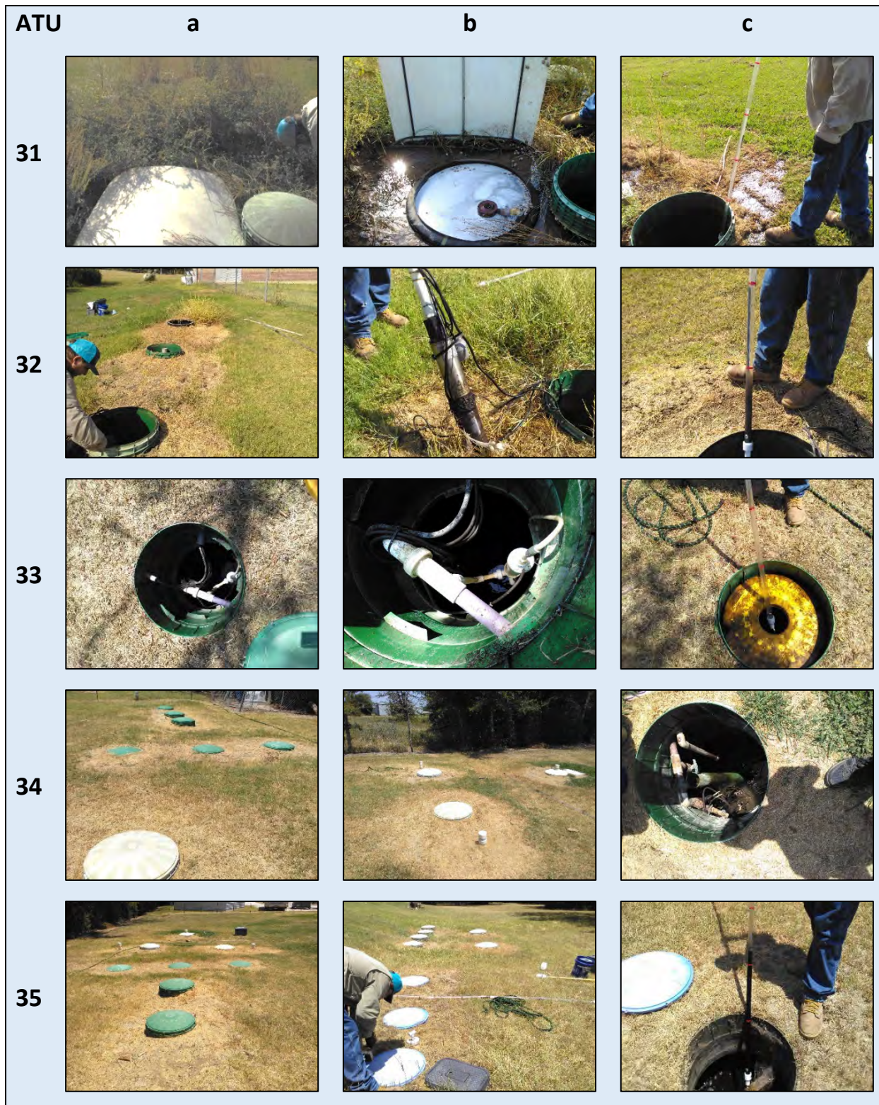
Plate 7. Photographs of ATU systems 31 through 35. Designations a, b, and c generally show a) overall system, b) pump tank, chlorinator, or lid condition or other anomaly, and c) sludge condition (if available).
