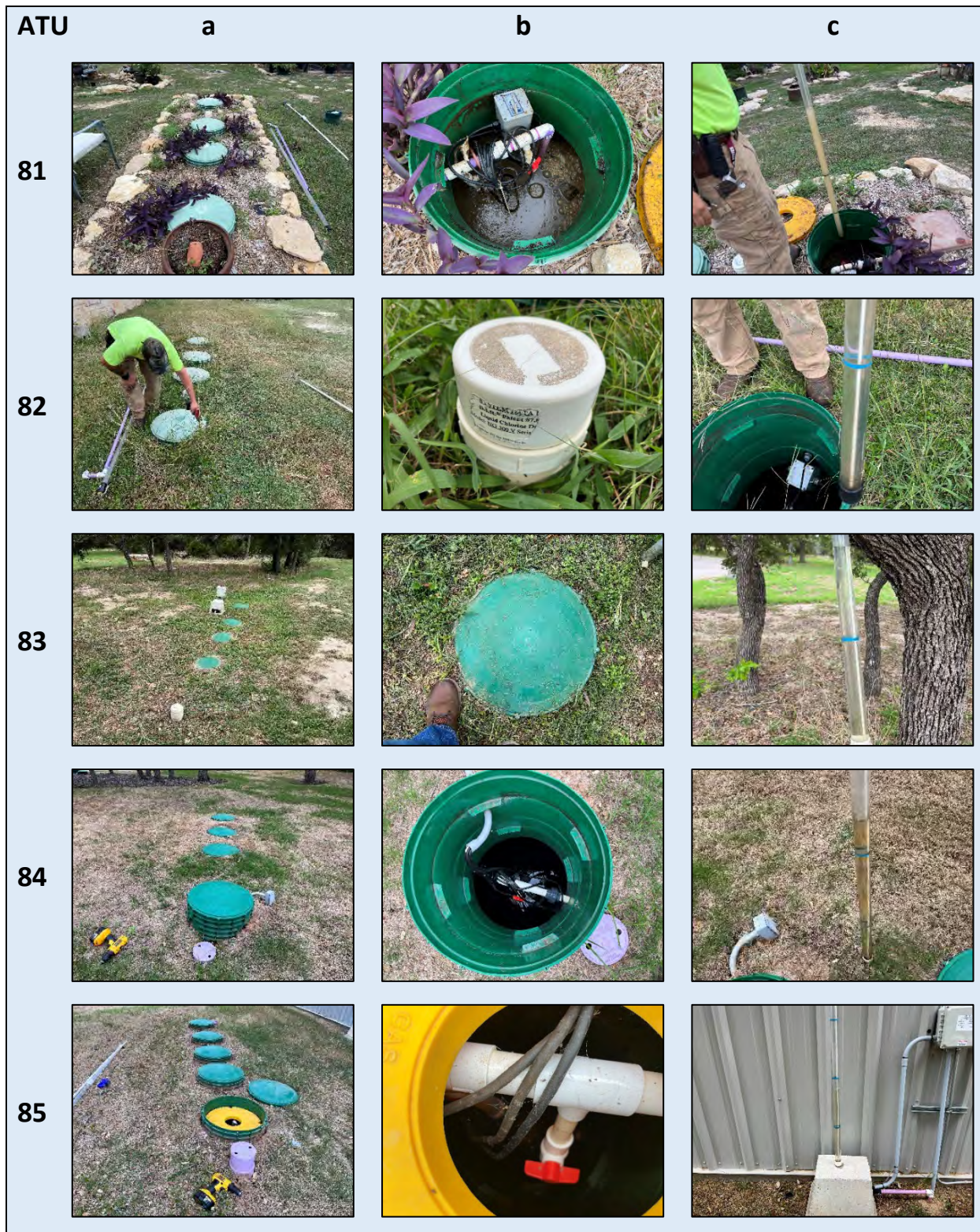
Plate 17. Photographs of ATU systems 81 through 85. Designations a, b, and c generally show a) overall system, b) pump tank, chlorinator, or lid condition or other anomaly, and c) sludge condition (if available).
