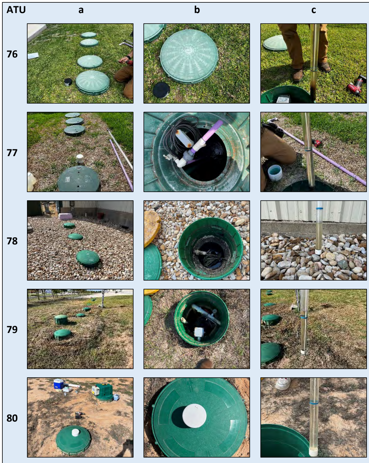
Plate 16. Photographs of ATU systems 76 through 80. Designations a, b, and c generally show a) overall system, b) pump tank, chlorinator, or lid condition or other anomaly, and c) sludge condition (if available).
