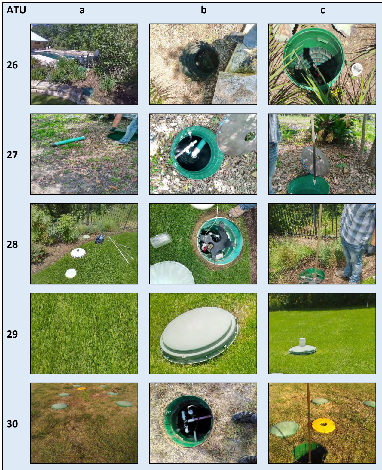
Plate 6. Photographs of ATU systems 26 through 30. Designations a, b, and c generally show a) overall system, b) pump tank, chlorinator, or lid condition or other anomaly, and c) sludge condition (if available).
